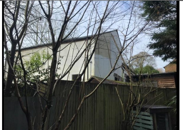
Photo 2 from front garden of Homestead to the 'Factory Building'
