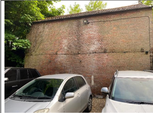
Photo 1 of existing flank of 10 Church Road
